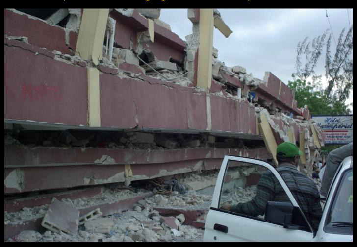
Here is an example of a somewhat better constructed building. More reinforcement was used partly because it was so open. Had it been solid walls, the reinforcement might have been leaner causing more pancaking as seen in the lower floor collapse.
