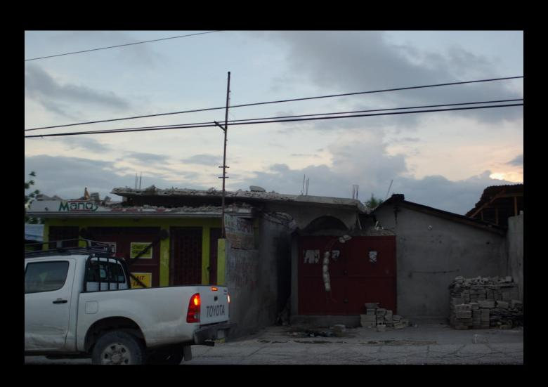
Bodies were trapped inside this former five story building. Lack of proper reinforcement ties between floor and walls may have contributed to this buildings total pancake. Had the walls and the floors been tied together, the building might have collapsed differently, forming triangle voids near the outside walls.
